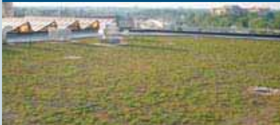
PECO Building, Philadelphia, PA
