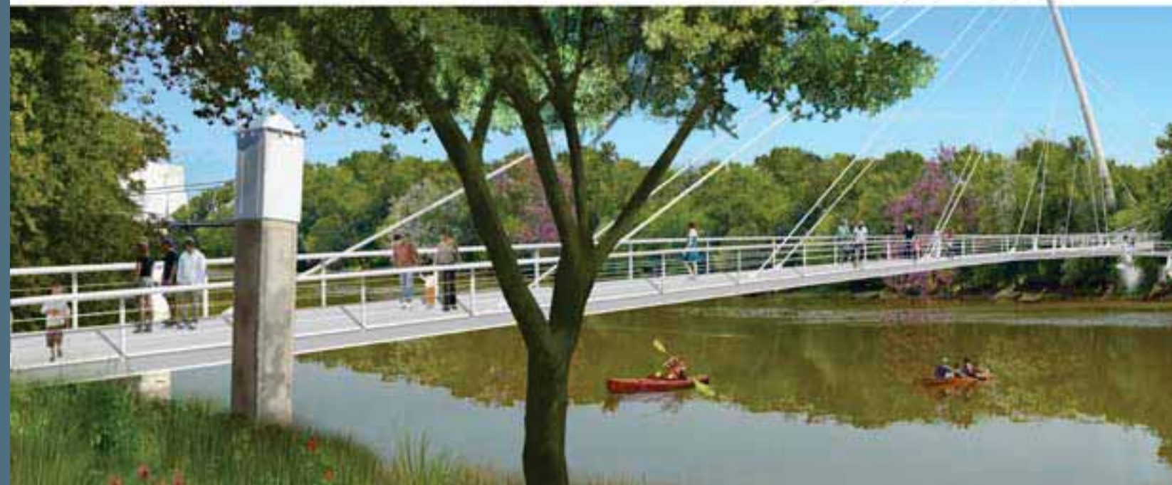
New pedestrian bridges across the Wabash are a key opportunity to create prominent civic symbols, demonstrating the engineering prowess and cultural interests of the community. The image shows a Cable Stay design bridge as an example of a design for the proposed Brown St. Bike/Pedestrian bridge. This design would eliminate the need for new bridge piers in the river. Image | WRT
