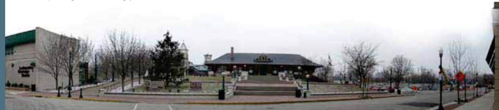
Riehle Plaza Existing Conditions. Image | Stanton Lambert
